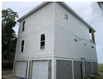
South east corner
