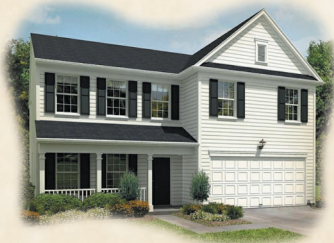
The Augusta Was $216,000 NOW $198,440 Ready June 09
